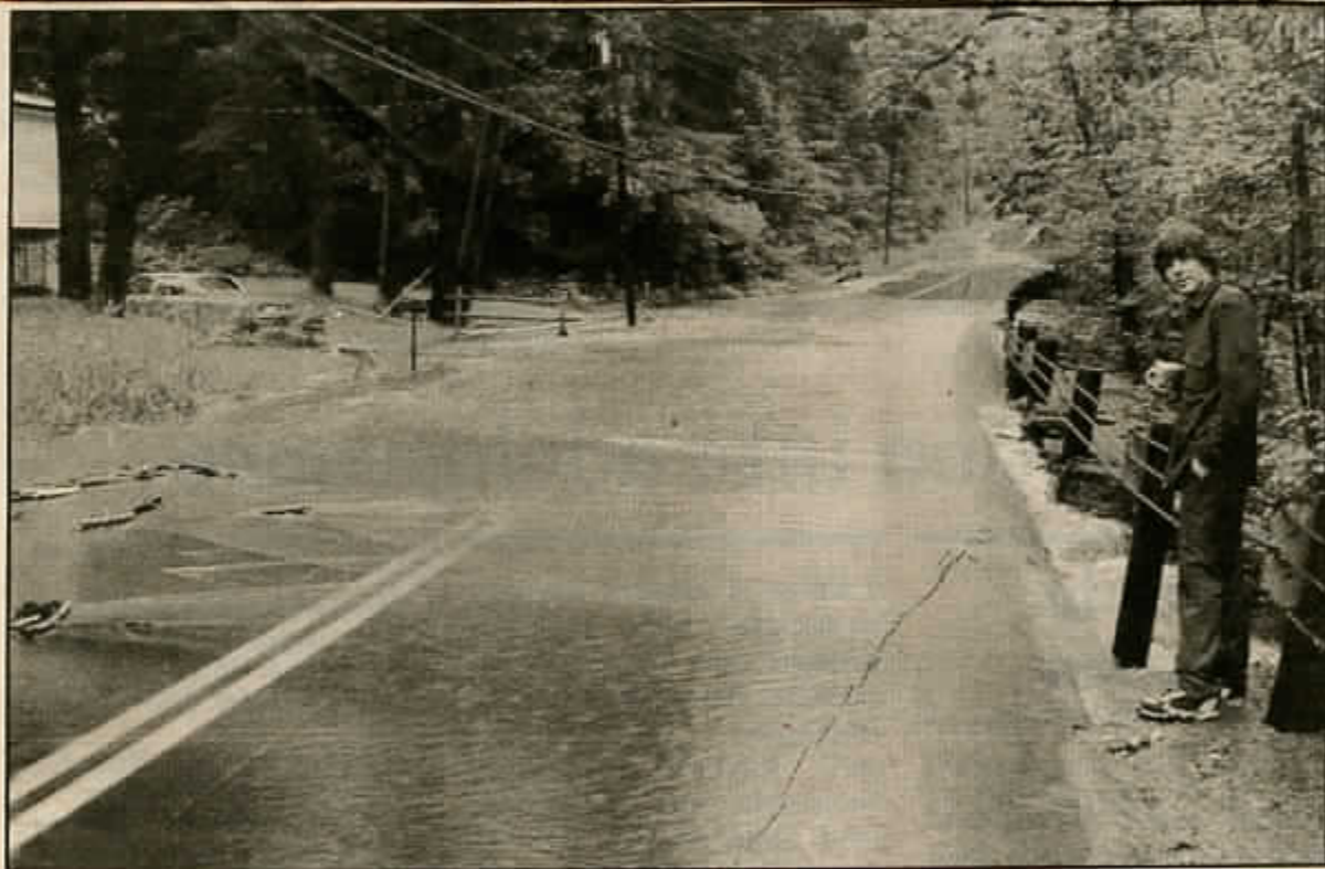
JUST HOW DEEP? — Cornish resident Bucky Demers stands near a neighbor's home on TownHouse Road in Cornish this morning, where water was flowing across the roadway following heavy rains. There were several reports of washouts and flooded roads in the Cornish area. (Wayne Carter photo.)
