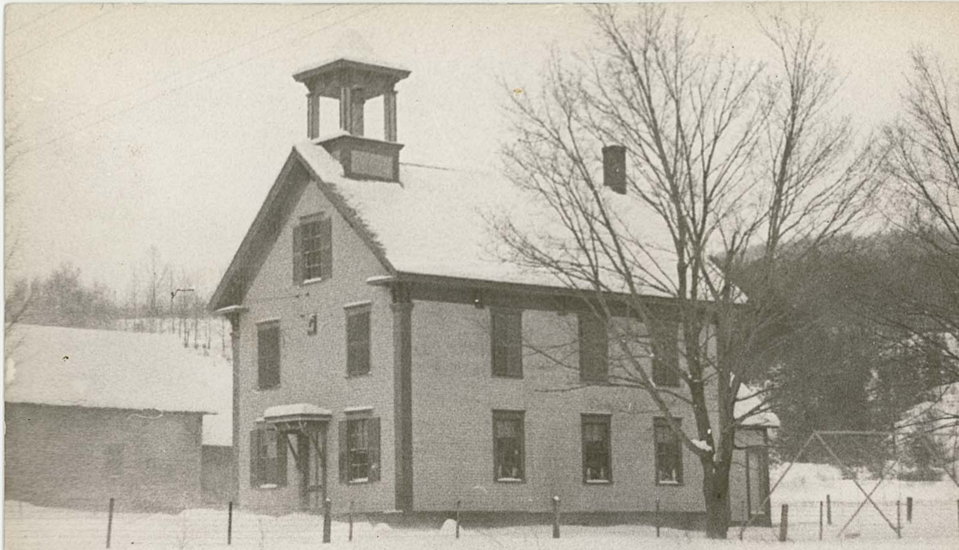
VILLAGE SCHOOL & MASONIC HALL - CORNISH FLAT NH
