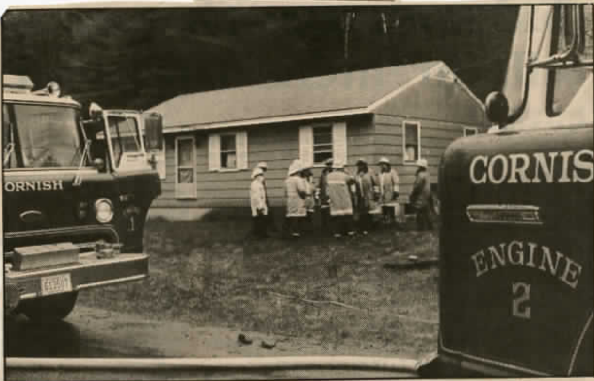
AN EARLY AFTERNOON fire Thursday damaged a single-story house on Center Road, Cornish. Valentina Ivanov and her son, whose name was not available, escaped without injury. Cornish Fire Chief John Rand suspects the cause of the fire was an electrical problem. The circuit breaker box was destroyed, and part of the floor in a bedroom had to be removed. "Structurally, there was not a lot of damage," he said. Cornish firefighters were assisted by five area departments. (Wayne Carter Photo)
