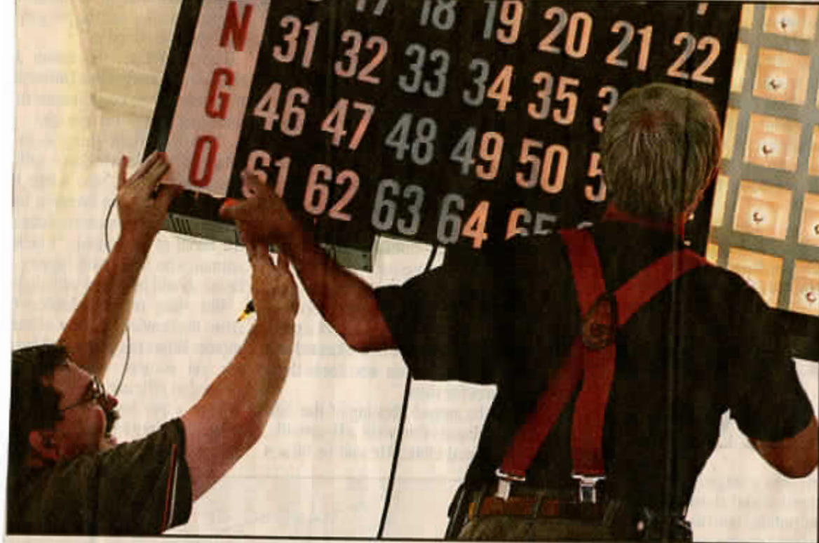
Cornish volunteer firefighters Mike Monette, left, and Bob Michal, right, slide the face of the bingo board together while replacing light bulbs and checking electrical connections before the fire department sponsored game at Cornish Town Hall. The state inspector paid a visit a week earlier and recommended the routine maintenance. The department has been running the game for the last four years.
