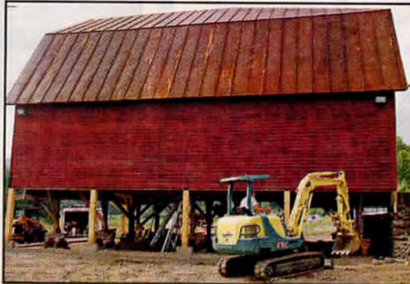
Organizers expect to complete the barn restoration in two years.
