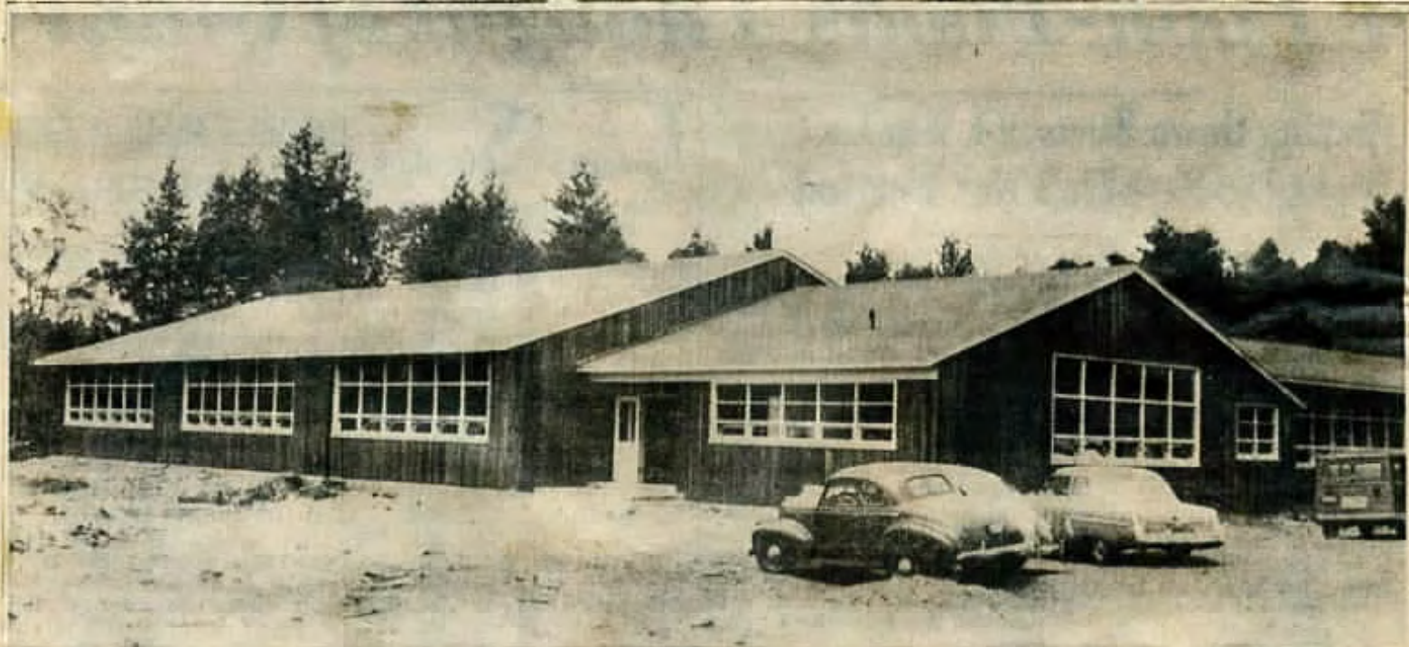
ONE INSTEAD OF SIX — The new Cornish school is nearing completion on the high ground adjacent to the town hall. The spacious, eight-classroom plant will replace six one-room schoolhouses that own neither central heating nor plumbing. The new building contains an assembly room, teachers' and utility rooms as well as the study area. Walls of the school are constructed of cinder block covered with wood sheathing. The MacMillin company of Keene is the contractor. Daily Eagle Photo—Titchen
