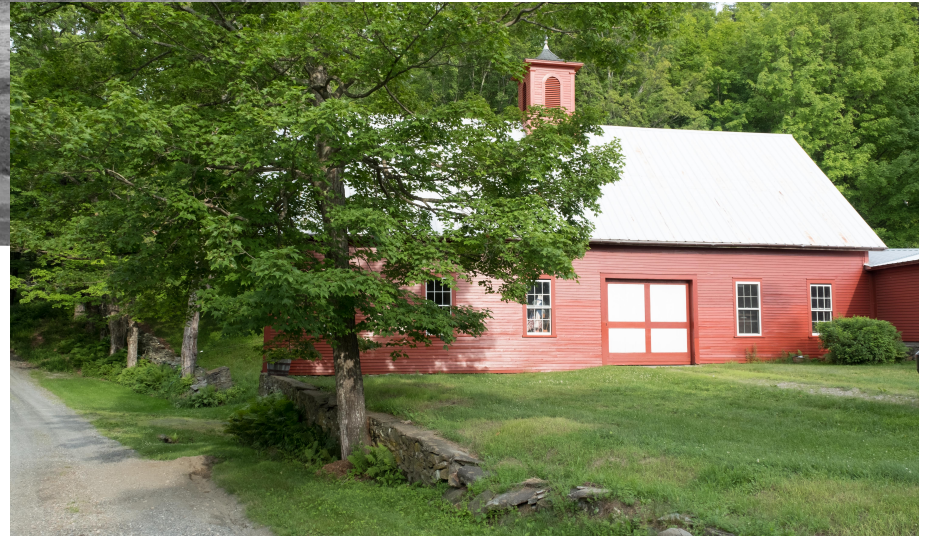
The black and white photograph (top) shows this cow barn during renovation. The original barn probably built in the late 19 th Century was converted to a horse barn in 1903 as it is today (lower photo).
