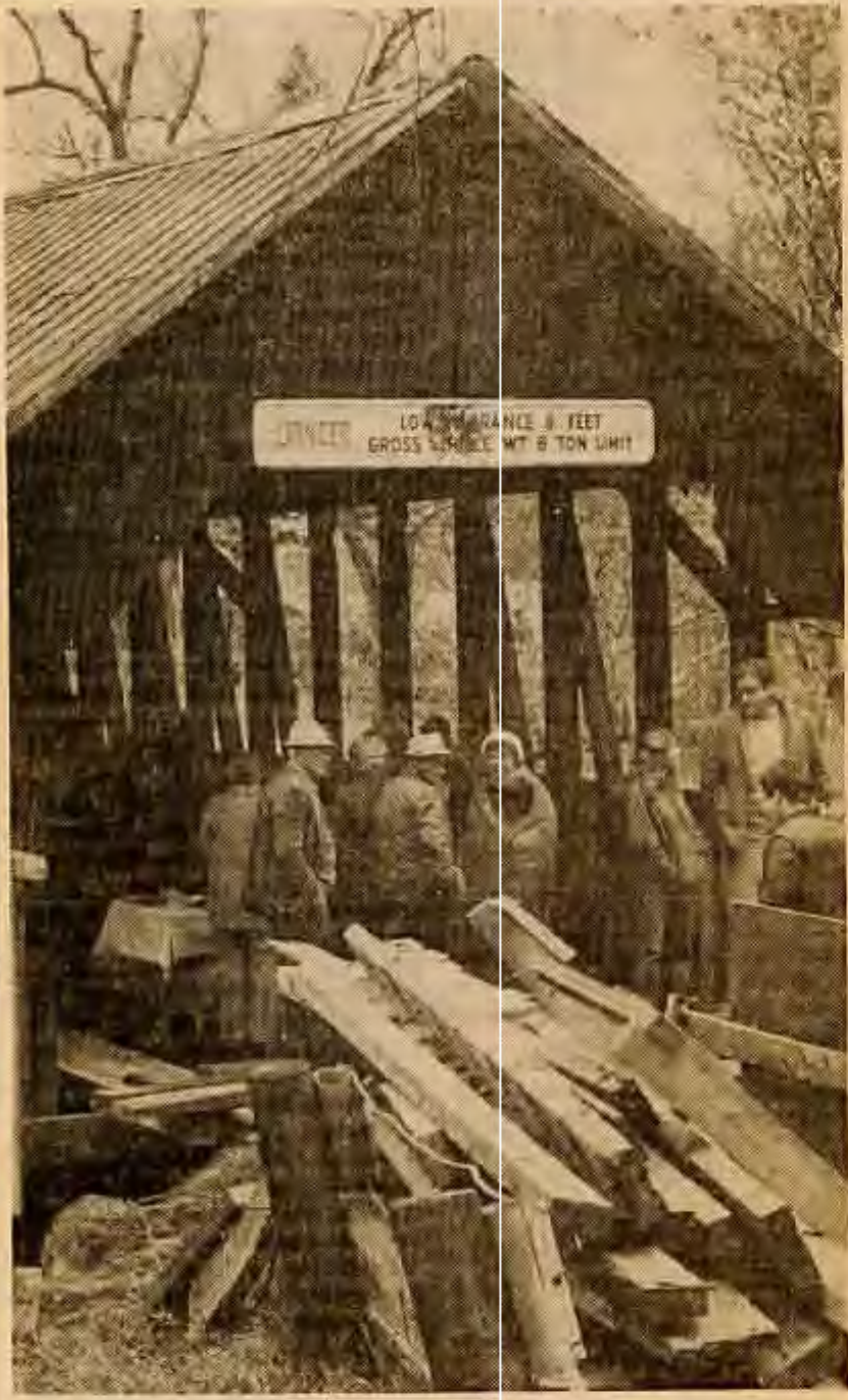
BRIDGE DEDICATION — About 50 people recently attended a dedication ceremony for the restored Dingleton Hill Covered Bridge, which spans Mill Brook in Cornish. The 101-year-old bridge was repaired by Milton S. Graton Associates of Ashland. It is one of four covered bridges in Cornish that were built by James F. Tasker in the 1800s. (Photo by Brad Hills)
