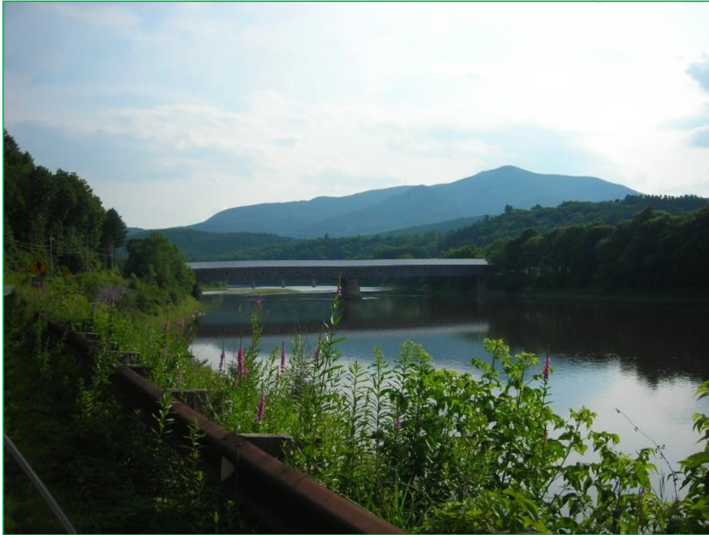
Cornish-Windsor Covered Bridge
