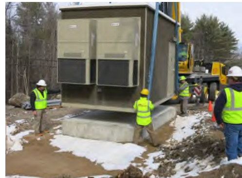
Electronis Hut being placed in Sandwich
