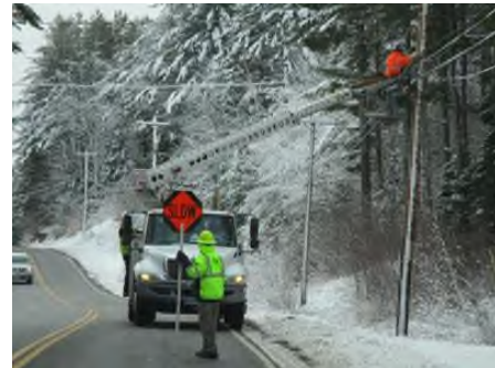
Building through the winter in Acworth
