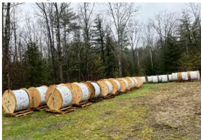
Spools containing 100 miles of fiber-optic line ready for installation in Sandwich, NH (April 2022)
