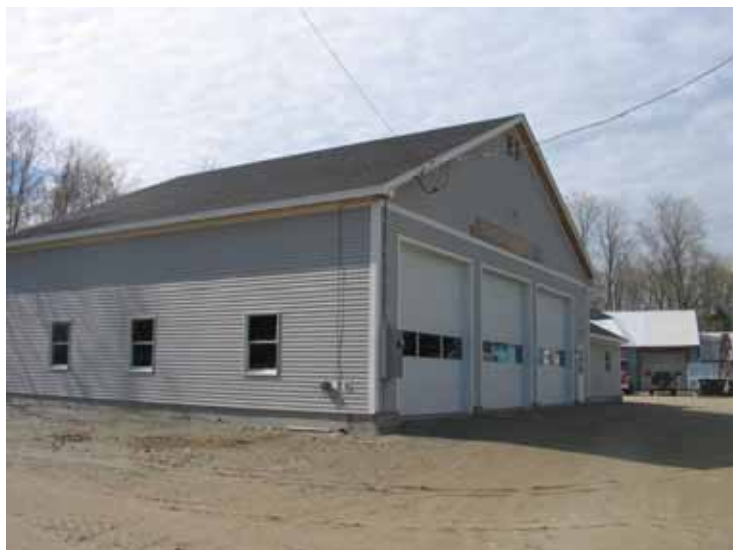
New (2008) Cornish Volunteer Fire Department station in Cornish Flat, constructed without taxpayer funds.
