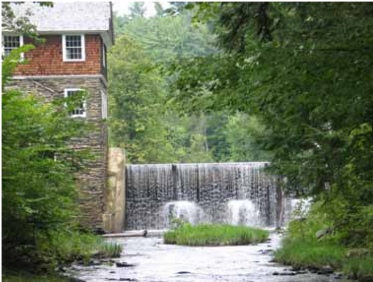
Blow-me-Down Mill, built in 1891 and restored by the National Park Service.
